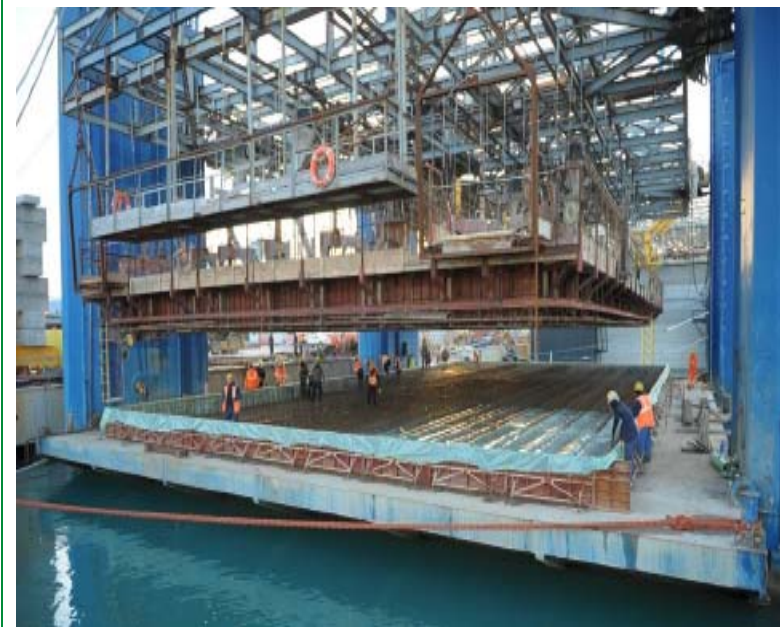
December 2012: building of the first REWEC3 caisson
